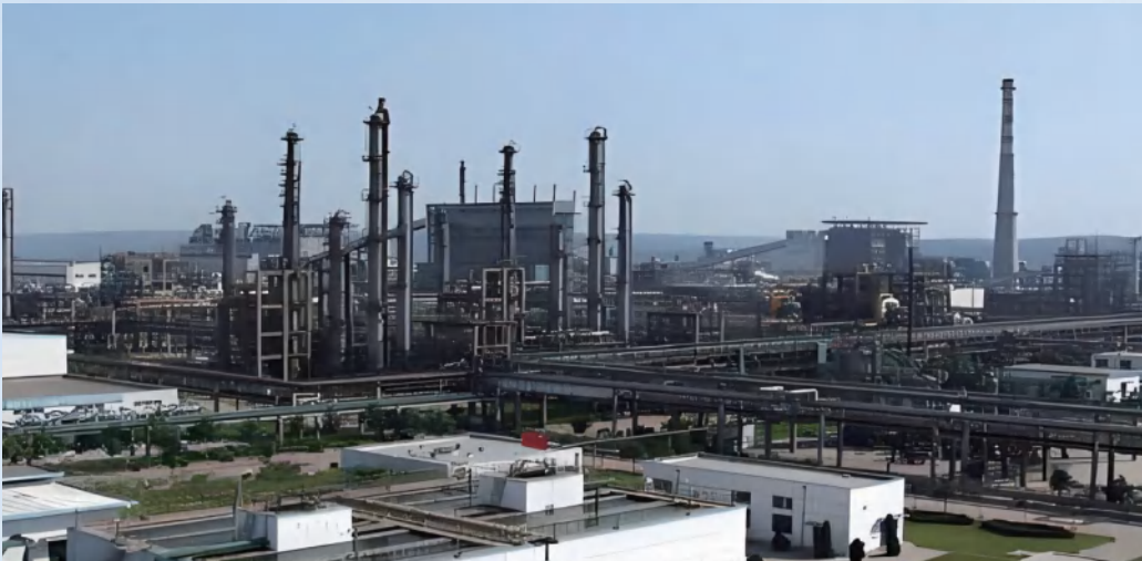
Air separation and compression
